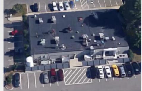
Odyssey's 10,000 sq. ft. wafer fabrication facility in Ithaca, NY
